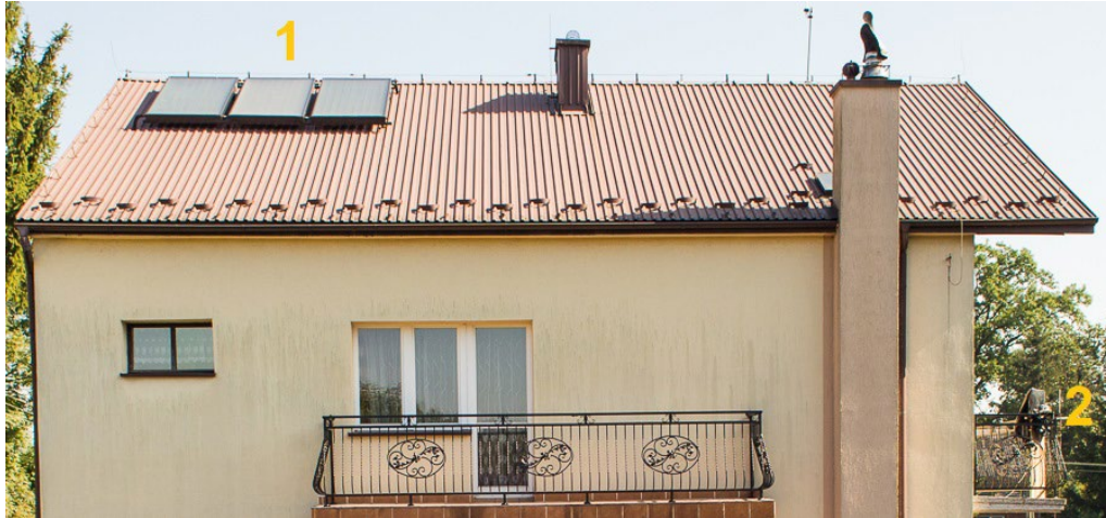
Fig. 2. Analyzed building with solar collectors (1) and solar radiation density meter (2). This picture shows the south-west side of the building
