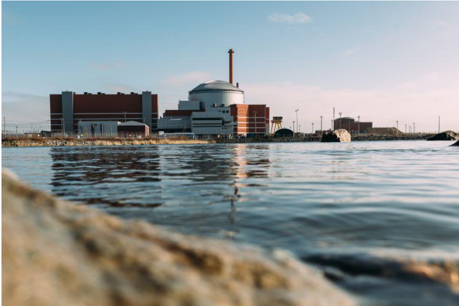
Fig. 6. Olkiluoto 3 Power Plant Source: (TVO 2023a)
